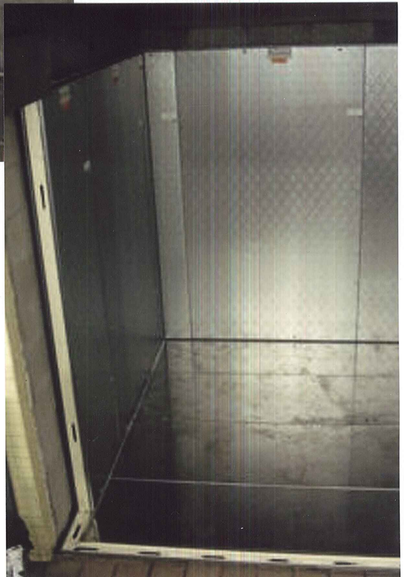
Set Wall Panels
