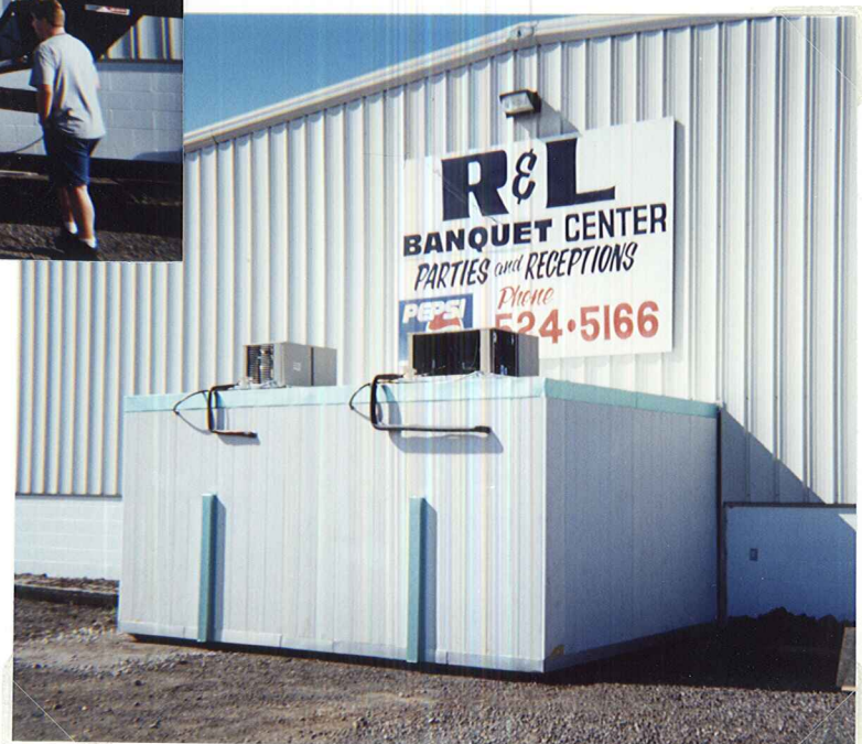
Delivery & Outside Installation of W.A. Brown Drop-off Walk-In Cooler
